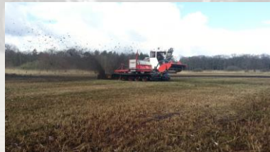
Tracked trench cutter
