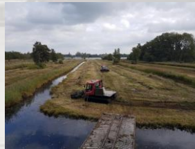
Tracked machine with pusher board
