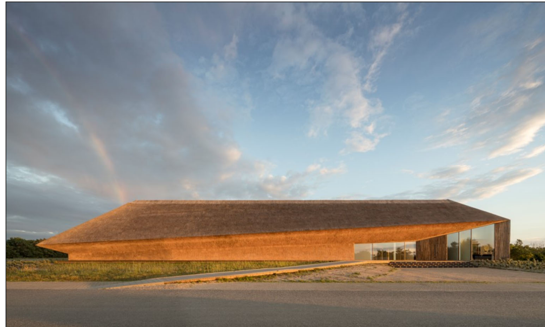
Reed thatched roof + walls (©Wadden Sea Centre, Ribe, DK)
