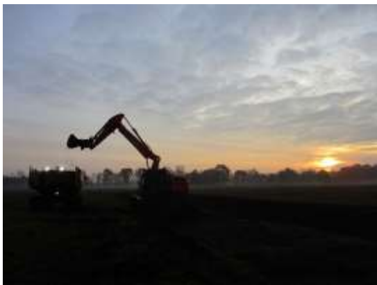
7 Starting top soil removal at Barver (Photo: J.-U. Holthuis)
