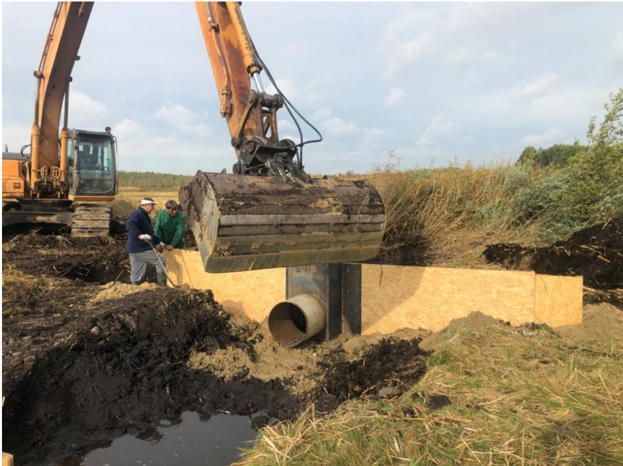
1 Figure installment of regulating dam in Žuvintas Biosphere Reserve in 2020 (Photo: N. Zableckis)
