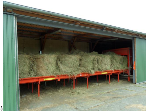
(a) Ruth Gregg and Deborah Land from “Natural England” (UK) learning about the district heating plant in Malchin, which is fired with biomass from rewetted fens. (b) shows the automatic feeding system for round bales and the disintegrating unit (photos: W. Wichtmann).
