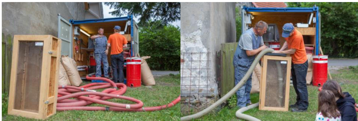
Isofloc-b' low-in machine in a container (left), first „blow-in test“ where results of filling the cavity (right)
