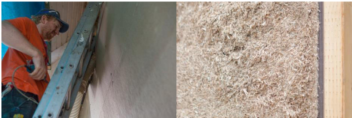
Preparing the wall for the test (left), the result: Typha blow in material after the test and after removal of the construction plate (right) (photos: T. Dahms)
